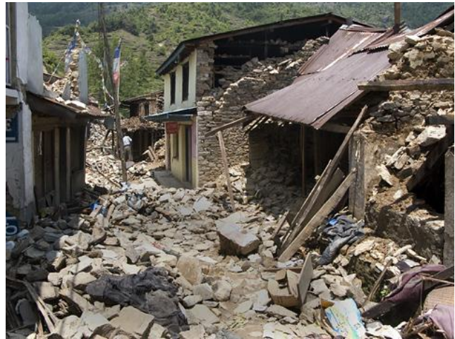
Village of Gul Bhanjyang in rubble
